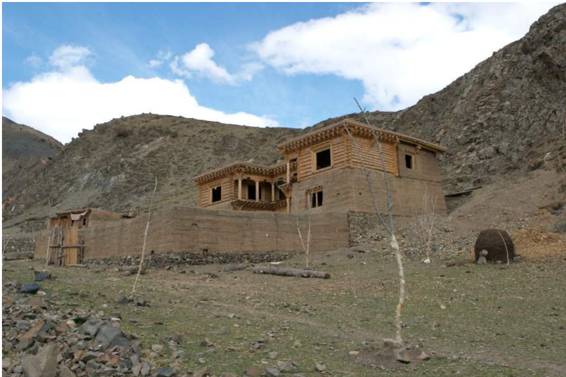
The school under construction in Rigul, Kham, Tibet. 2006
